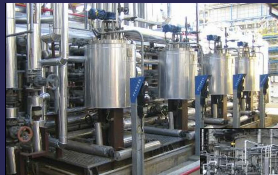
ACR feed filter for CR-40 DAO GOFINER Unit (Deasphalted Oil) Priolo Gargallo, Italy
