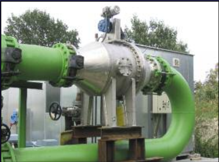
AISI 316L stainless steel SACIL filter for sea water. Fusina, Italy.
