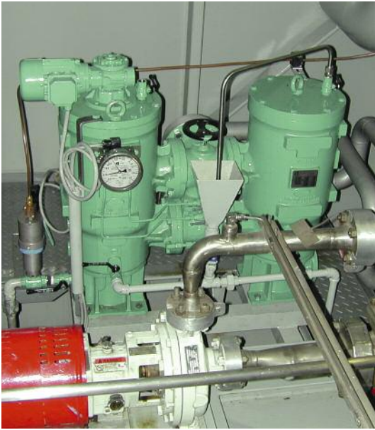
Booster System - Gas Turbine GE LM 2500 Ship "JEWEL OF THE SEAS" DACXT Filter - Filtration 10 µm absolute
