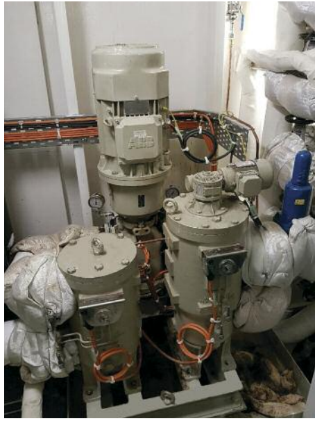
Supply System - Diesel Engine MAN 14 V48/60 Ship "CARNIVAL VISTA" ACT Filter - Filtration 10 µm absolute
